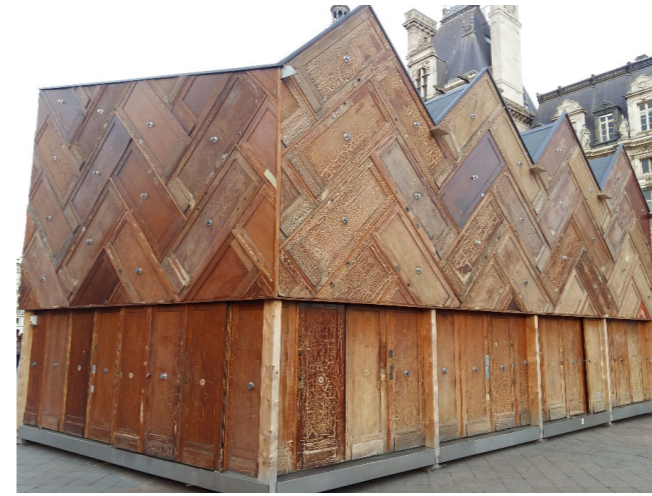
Figure 4. Circular pavilion in Paris made of recycled doors
