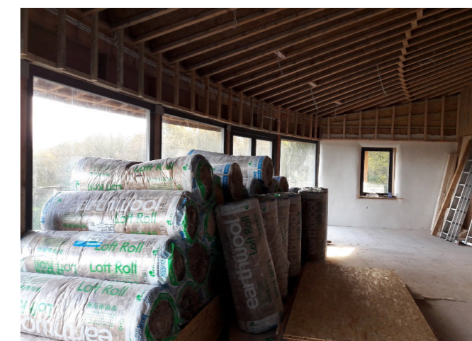
Figure 2. Natural materials used for building insulation – Curden Valley Park Visitor Centre
